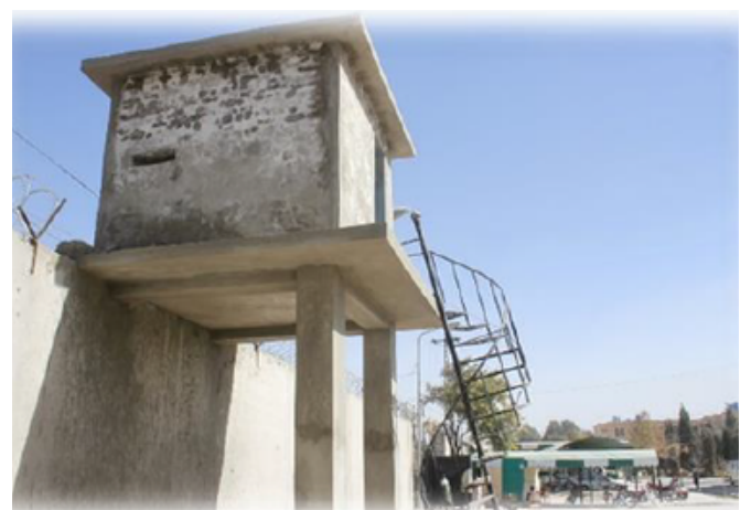
Pictures of newly constructed front watch towers at NIPA Quetta.
