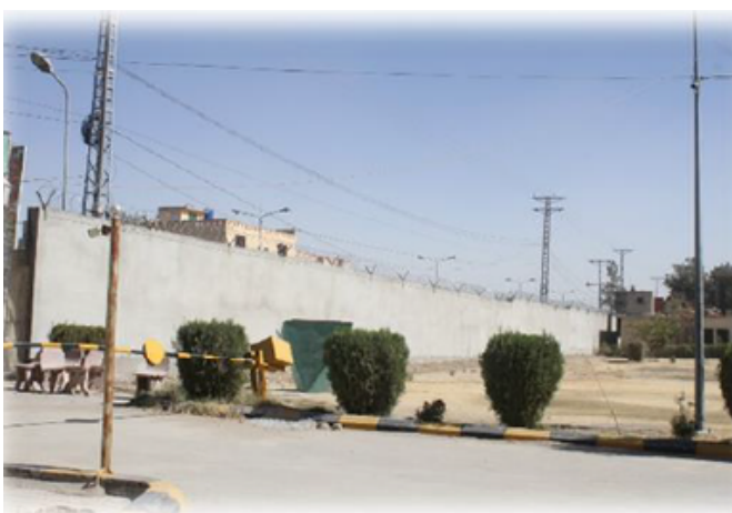
Pictures of newly constructed front boundary wall at NIPA Quetta.
